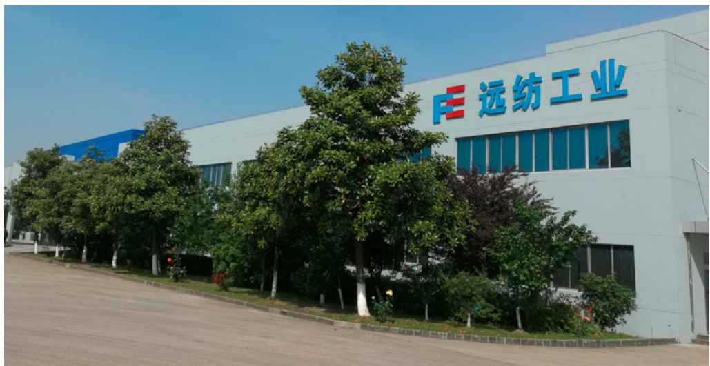
Front view of the Far Eastern Industrial factory, Wuxi
