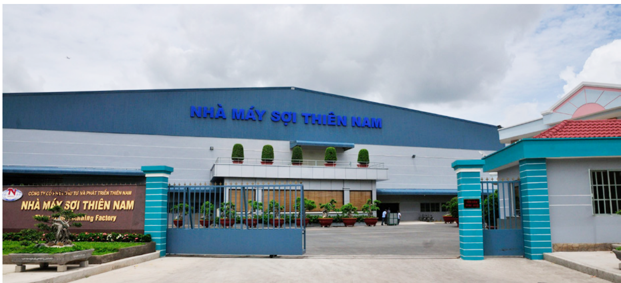
Entrance to factory Thien Nam
