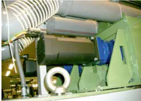
Fig. 8 - Installation of new motors
