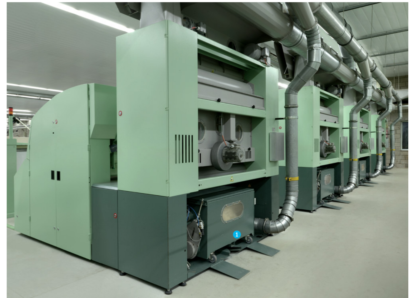
Separate licker-in waste disposal 1 connected to the centralized waste collection plant.
